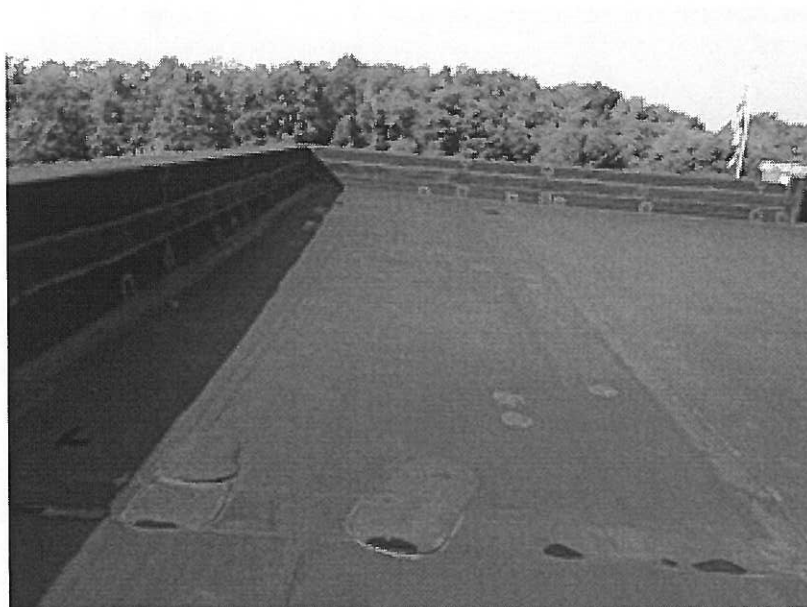
Image 2. Overview continued. The new wall flashing will extend up and over the walls, and with new metal edge installed.
