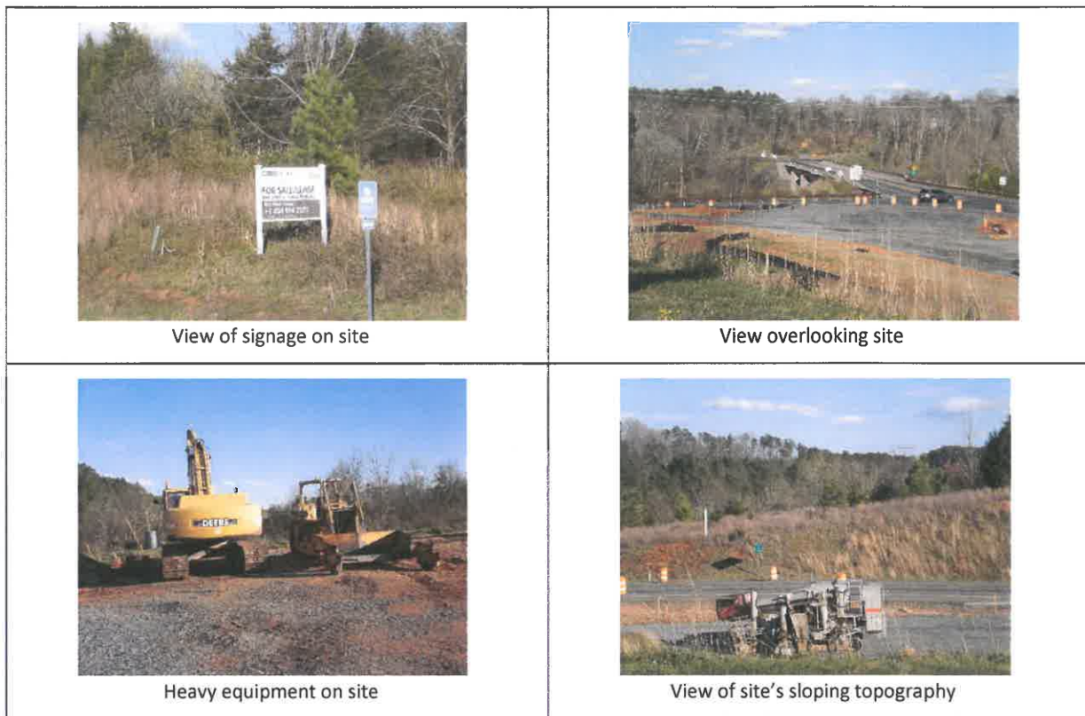
Figure 8 Views of Future Business Park (Site 3)
