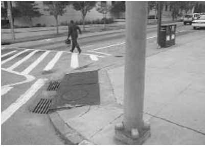
A curb cut located outside Atlanta's City Hall. The location of the sewer grate makes it almost impossible for a mobility impaired individual to cross the street.
