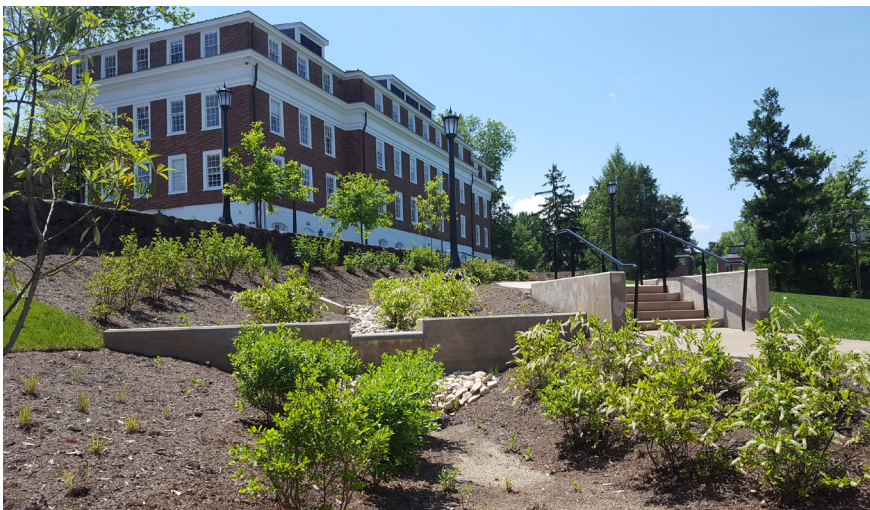
O'Neil Hall Renovation
