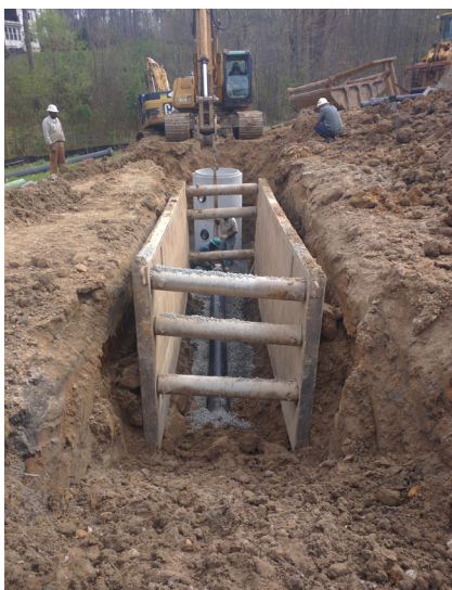
Rivergate Pump Station
