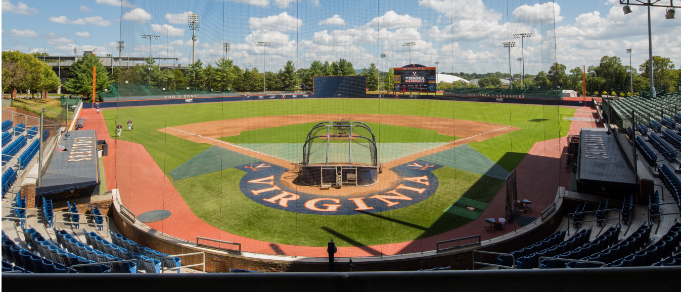
Davenport Field Renovation
