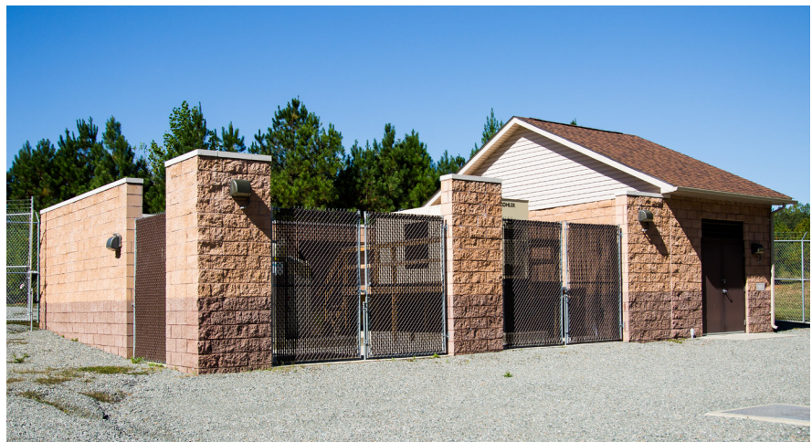
Grassy Swamp Wastewater Pump Station
