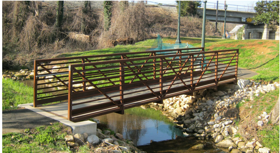
Lambeth Pedestrian Bridge
