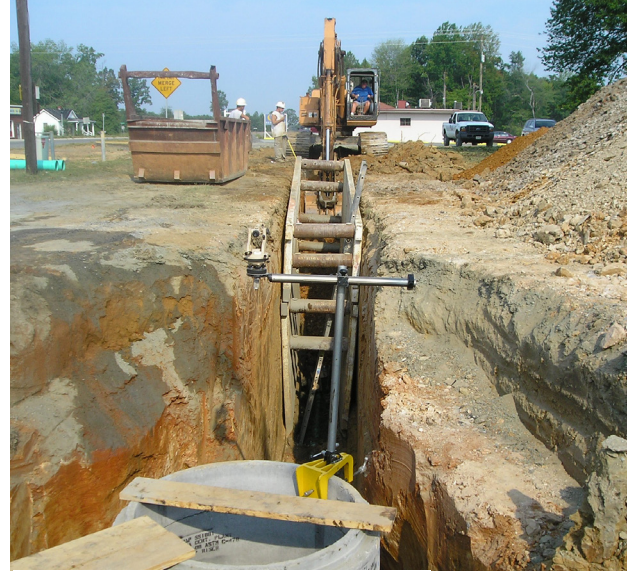
Zion Crossroads Sewer Improvements
