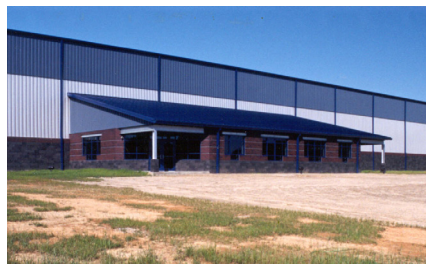
Ringgold East Industrial Park
