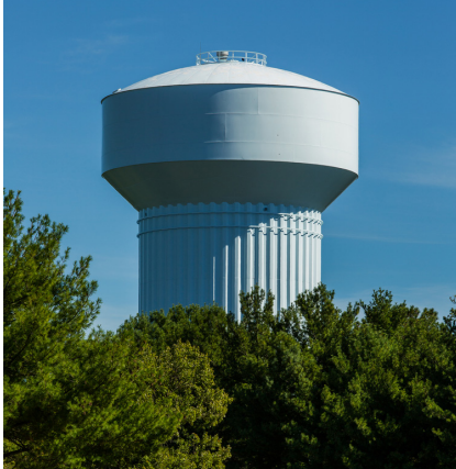
Creighton Elevated Tank
