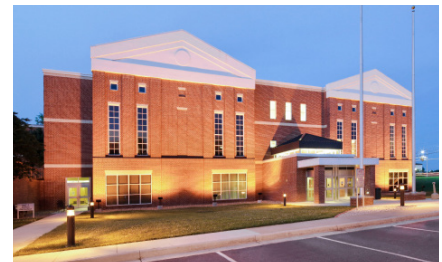
Campbell County Government Office
