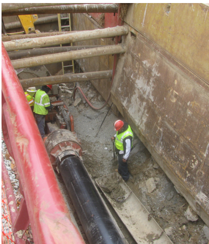
Cedar Lane Waterline
