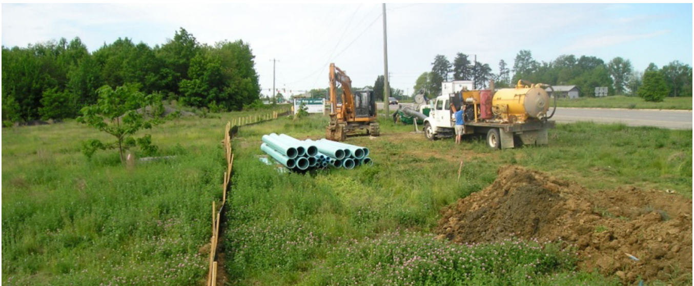
Water System Improvements
