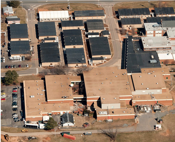
School Earthquake Assistance
