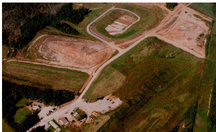
Pittsylvania County Landfill
