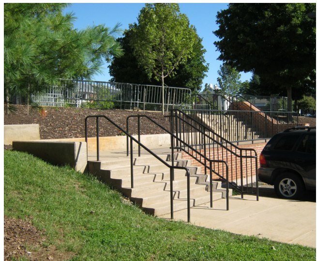
Arlington Boulevard Improvements
