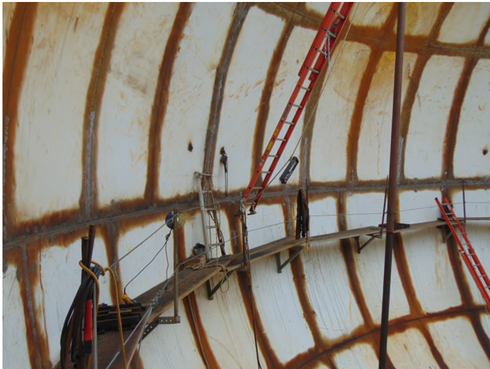
Photo #: 14 Description: Interior Wet: View of S1, S2, S3, & S4 courses.
