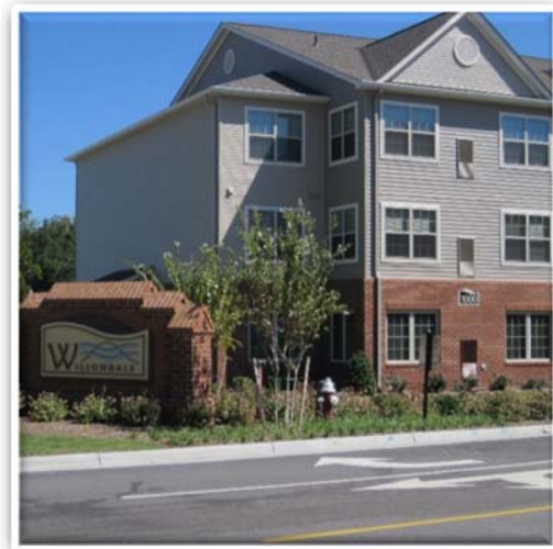
WILSONDALE Hampton, VA Completed 2011 Mixed Use/Mixed Income Development 150 Affordable Apartments 60 Luxury Apartments 11,000 s.f. Retail & Commercial Space Total Development Cost - $25.0 Million
