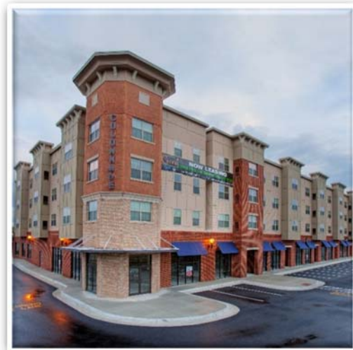
COLONNADE AT ROCKTOWN Harrisonburg, VA Completed 2010 Mixed Use/Mixed Income Development 60 Affordable Apartments 6 Luxury Apartments 24,000 s.f. Retail & Commercial Space Total Development Cost - $10.0 Million
