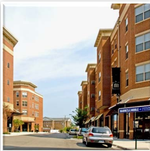
MID TOWN SQUARE Farmville, VA Completed 2006 420 Student Beds- Longwood University 44,000 Square Feet of Retail & Commercial Space Total Development Cost - $25.0 Million
