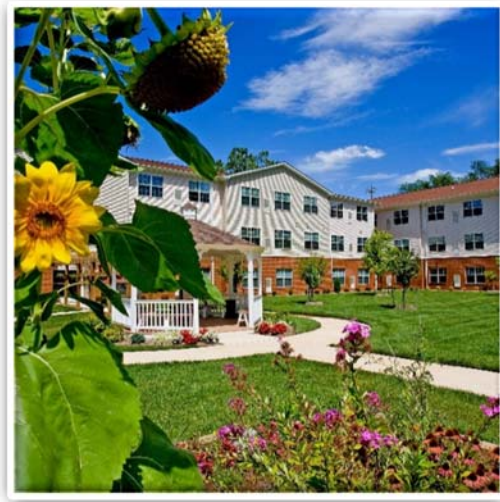
MOFFETT MANOR Warrenton, VA Completed 2007 98 Affordable Senior Apartments Total Development Cost - $10.5 Million
