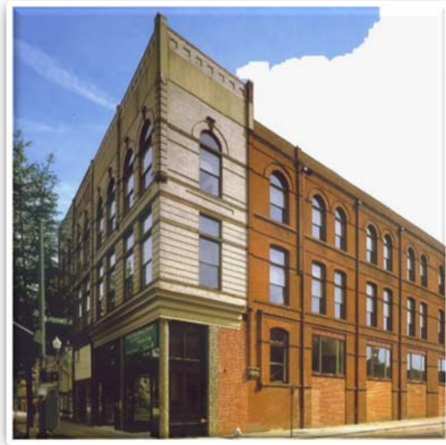
ONE EAST BROAD ST Richmond, VA Completed 1999 Historic Adaptive Re-Use 19 Luxury Apartments 6,500 Square Feet of Commercial & Retail Space Total Development Cost - $1.8 Million
