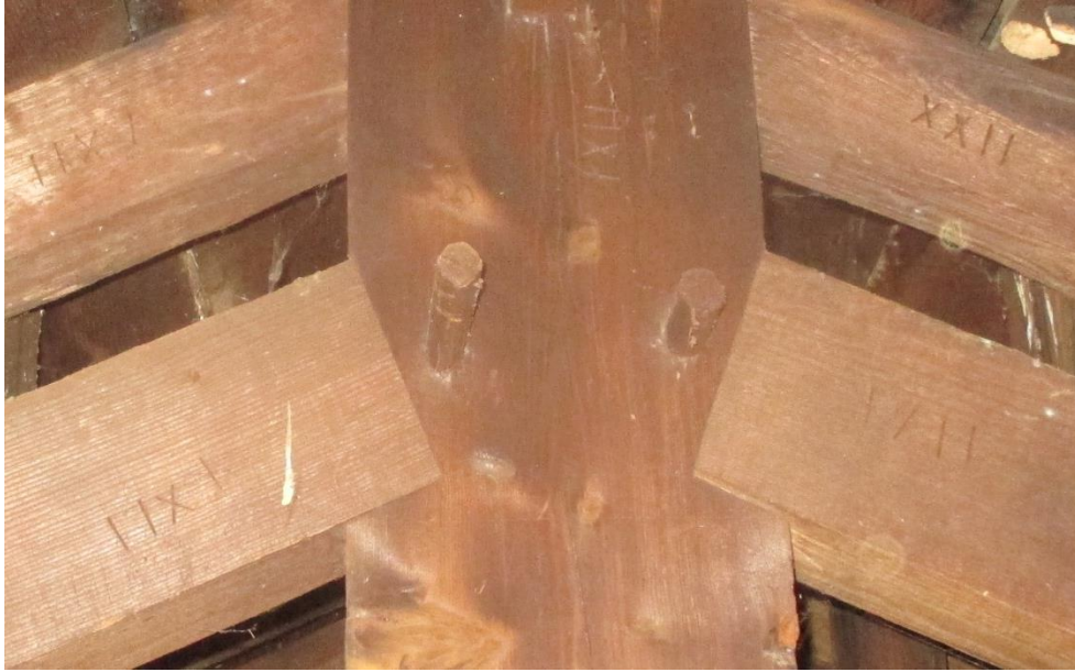
Figure 59. Detailed view of fabrication markings on roof trusses for use in assembly
