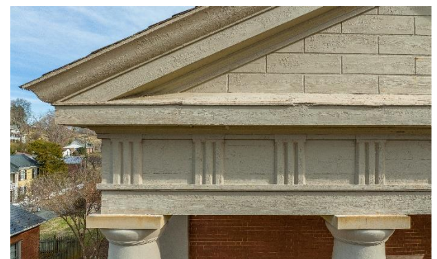
Figure 28. Portico entablature detail
