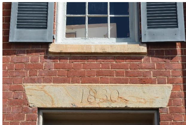
Figure 30. Detail of stone sill and lintel
