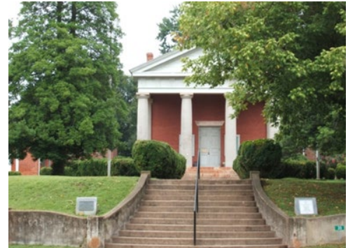
Figure LU-21, Historic Courthouse
