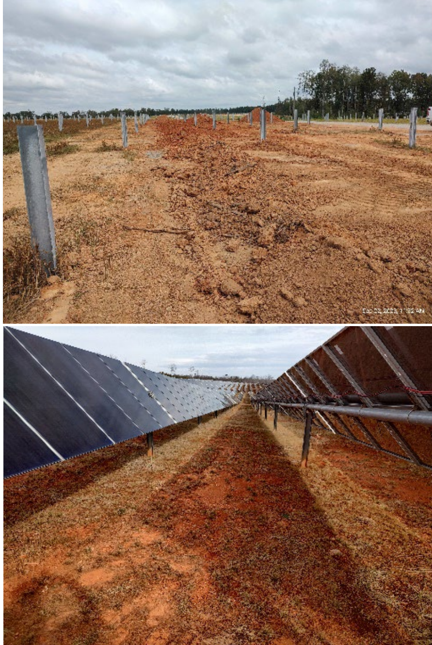
Figure 1. Utility-scale solar (USS) facilities during initial stages of development and stabilization in the Virginia Piedmont. During the initial establishment phase (top) trenching, cut/fill and grading activities will disturb anywhere from 15 to > 75% of most sites. Once final grading is completed and infrastructure is installed (bottom), full revegetation and stabilization against erosion losses generally takes several years. In general, revegetation practices should result in \geq 75\% living perennial cover of the intended or other appropriate species, which are most commonly mixed grass/legume stands. Note the “drip line” evident below the panel edges.
