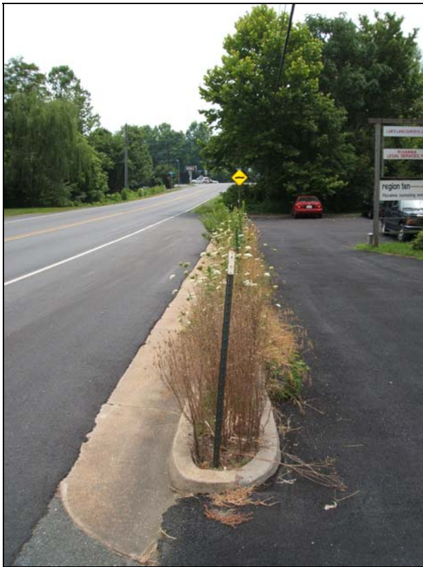
The existing access management of Rt. 15 should be improved with a coordinated plan of curb and gutter, clear driveway and pedestrian zones, and other devices.
