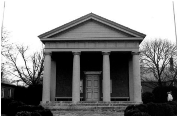
Figure HP-2, Historic Courthouse
