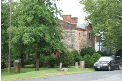
Figure LU-19, Old Stone Jail
