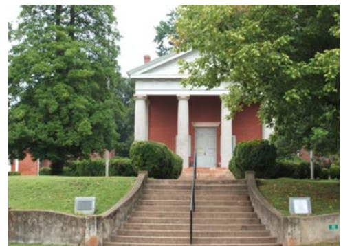
Figure LU-21, Historic Courthouse
