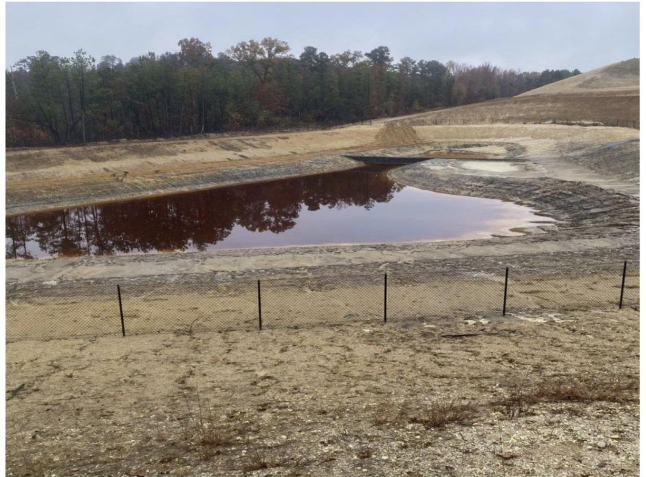
Figure 5. Exposure of acid sulfate soil (ASS) materials in a deep stormwater pond excavation in Miocene age Coastal Plain sediments in the Fredericksburg area. The darker gray sulfidic materials are reduced (anaerobic) and then oxidize to form sulfuric acid and very low pH (< 3.5) and metal enrichment (Al, Fe and Mn) in soil and receiving waters. Remediation of these materials requires very heavy lime applications (> 15-50 tons ag lime per acre six inches).
