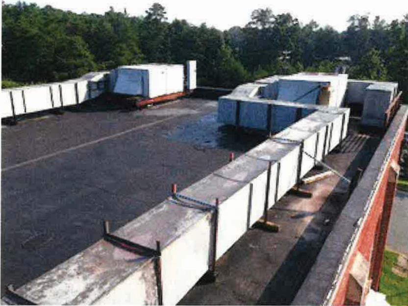
Overview of Performing Arts Roof.
