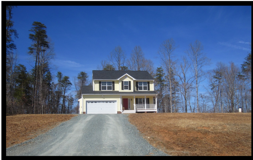
Image 4: A new single-family home under construction in the Boxwood subdivision.
