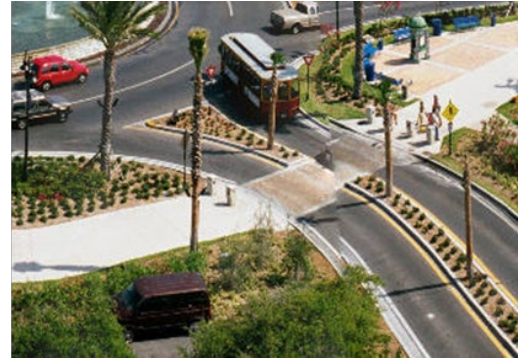
Figure LU-15, Median splitter islands and set-back crosswalks
