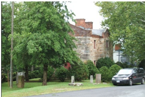
Figure LU-19, Old Stone Jail
