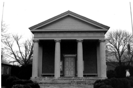
Figure HP-2, Historic Courthouse
