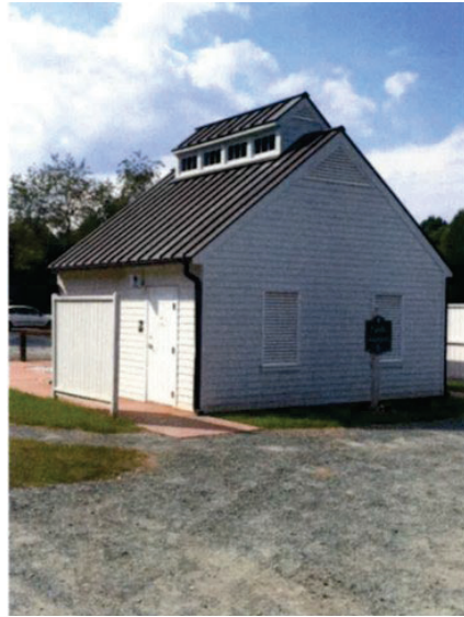
PG Bathrooms (plan is to add about 1/3 more inside facilities)
