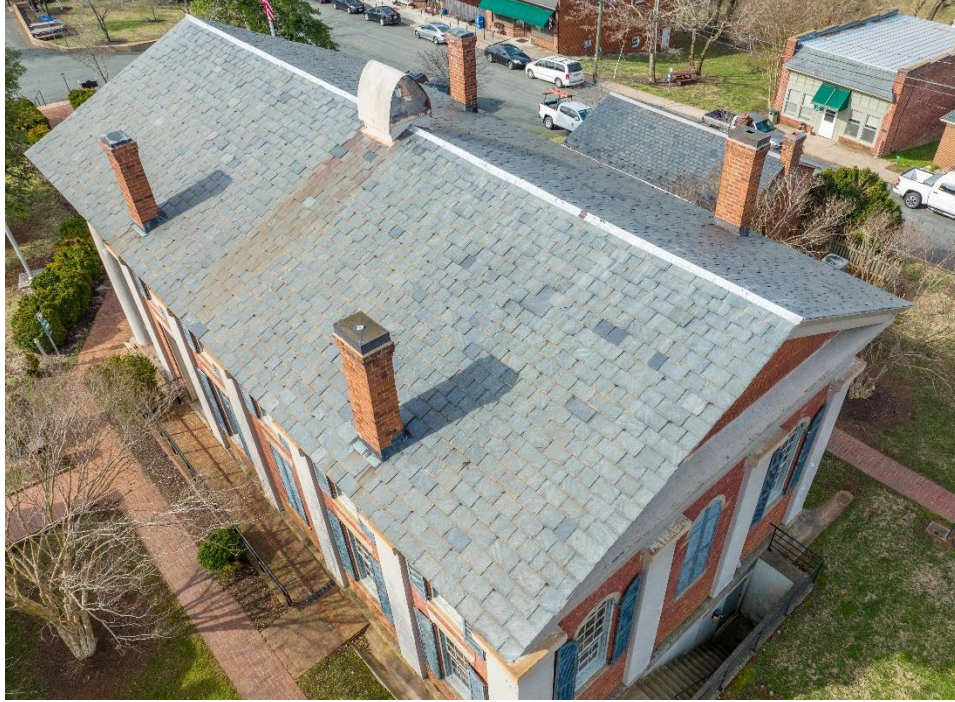
Figure 33. View of roof
