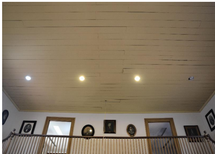
Figure 45. View of courtroom ceiling
