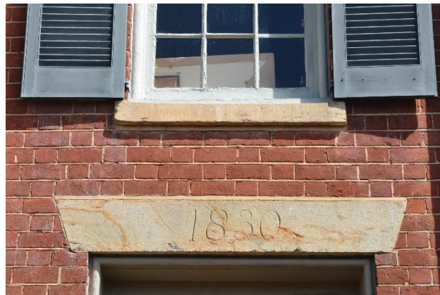
Figure 30. Detail of stone sill and lintel
