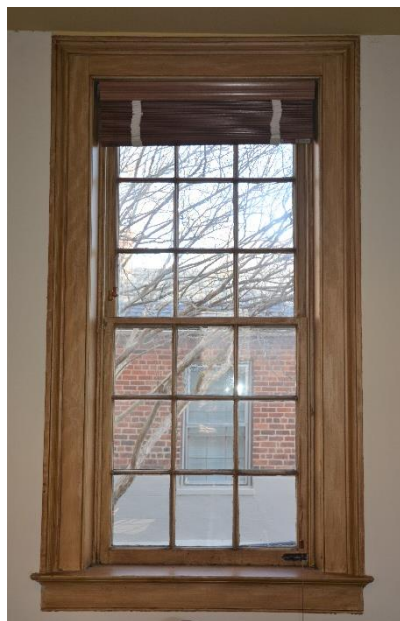
Figure 43. View of typical window
