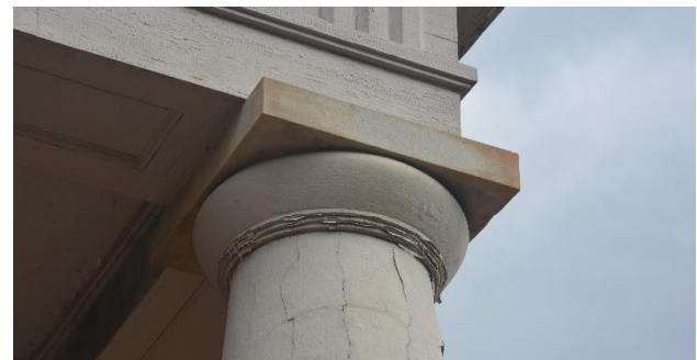
Figure 27. Column capital detail
