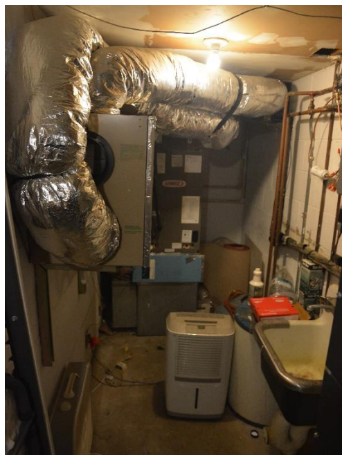
Figure 54. View of basement mechanical room
