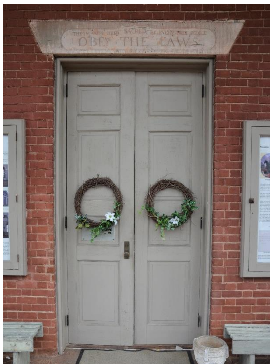
Figure 31. South entrance doors
