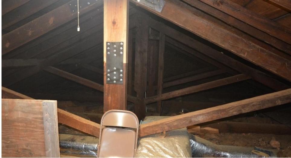
Figure 57. View of roof structure with repaired truss in foreground
