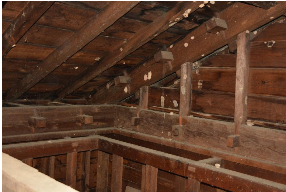
Figure 58. Detailed view of roof structure at southeast corner of portico
