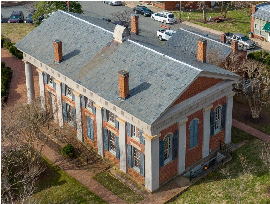
Figure 56. Aerial view of building from northeast
