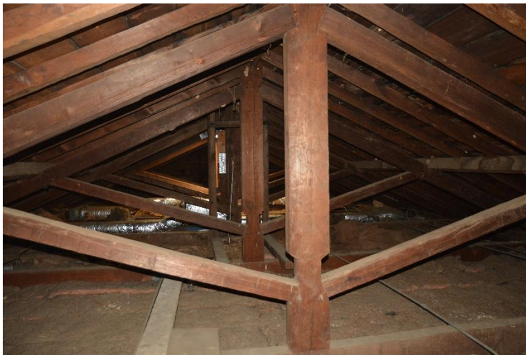
Figure 50. View of attic to south
