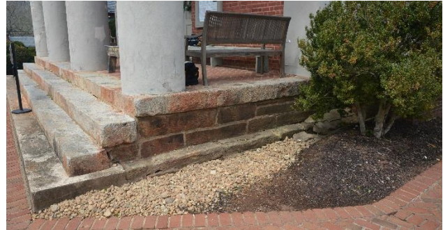
Figure 25. Portico floor and stairs
