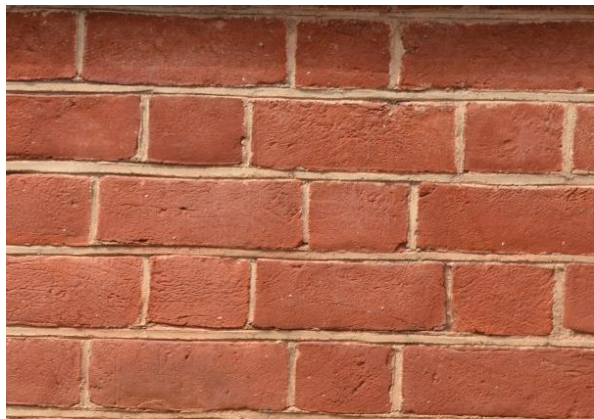
Figure 29. Detail view of brick wall
