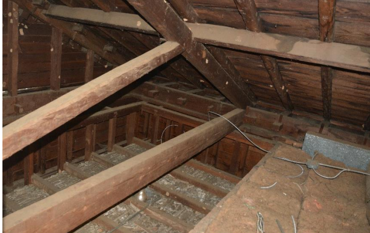
Figure 51. View of south end of attic above portico ceiling
