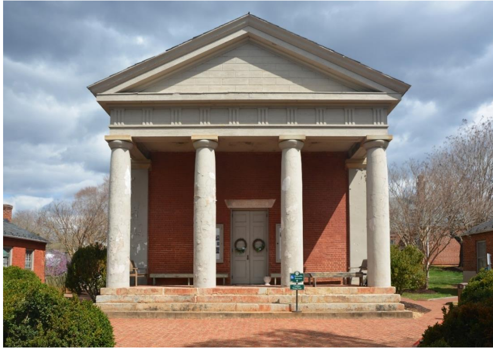
Figure 1. South Elevation of Fluvanna County Historic Courthouse
