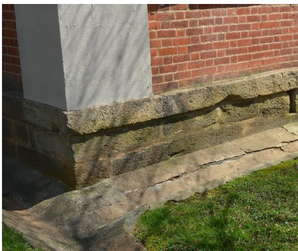
Figure 24. Detail view of foundation
