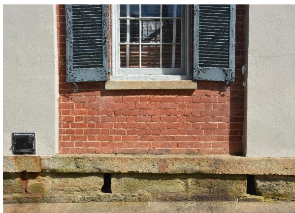
Figure 23. Detail view of exterior wall
